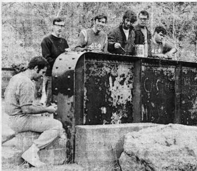
"... scraping and painting the graffiti-covered steel bridge that spans the public highway."
