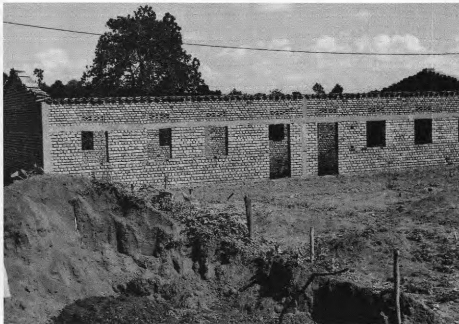
Burundi Yearly Meeting's new conference center under construction
